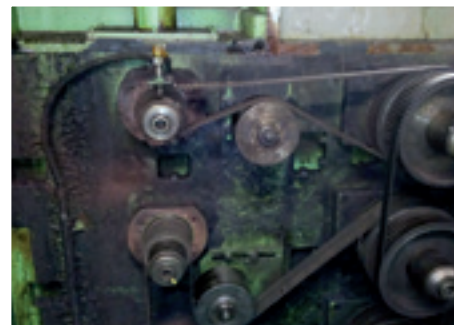
Fig. 3. Belt drive before reconditioning.
