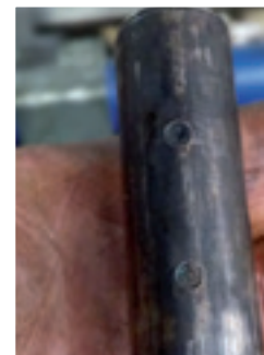
Fig. 5. Spray pipe when dismantling the pipeline
