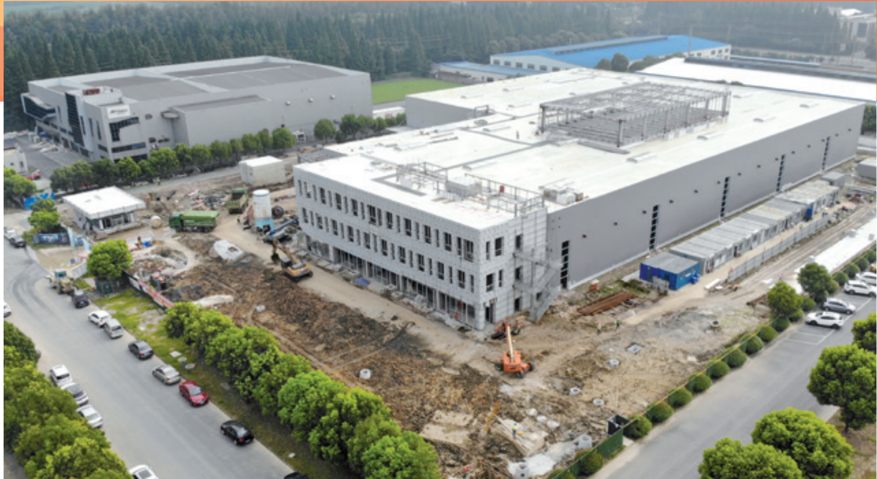
Fig. 1. The construction works on the new NMC factory are progressing well.
